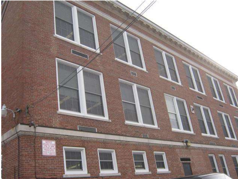
Exterior masonry bearing walls looking at east face
