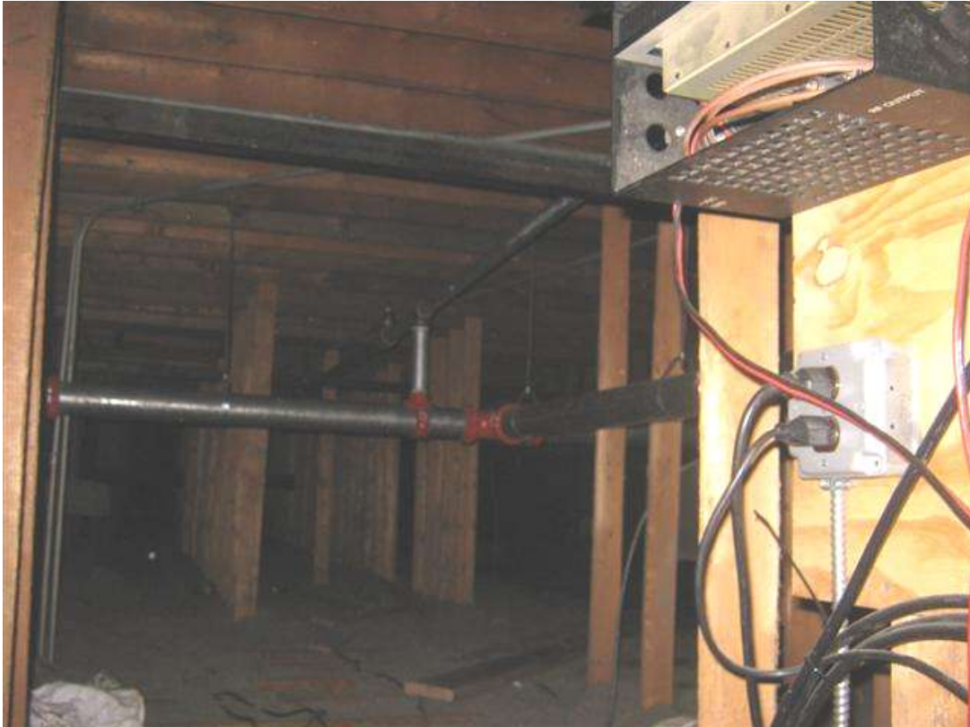
Bearing stud walls throughout the attic space
