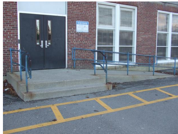
Northeast entrance and ramp
