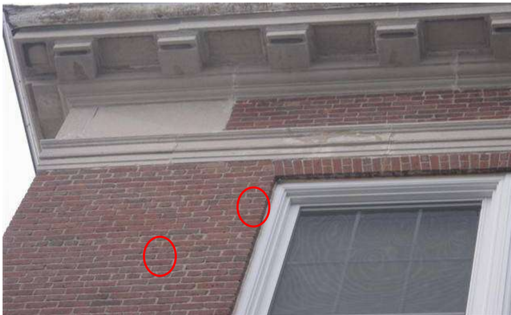
Spalled bricks
