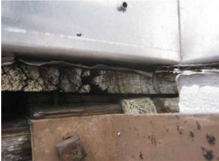
Tongue and groove wood roof deck at hatch
