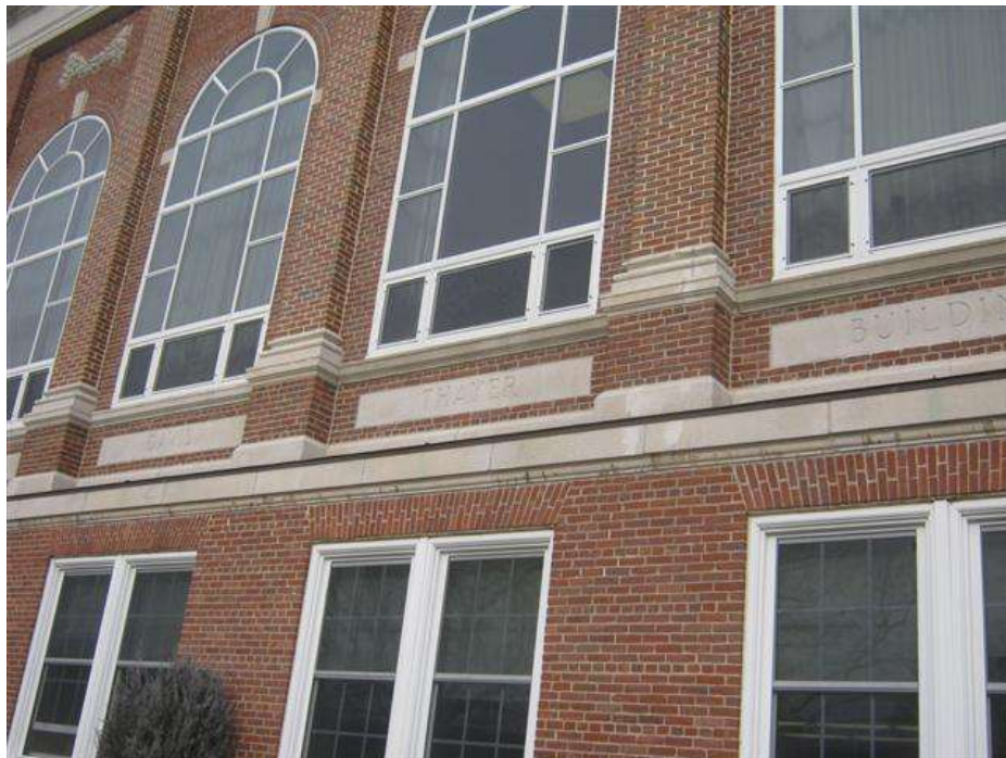
Exterior brick wythe viewed along south wall
