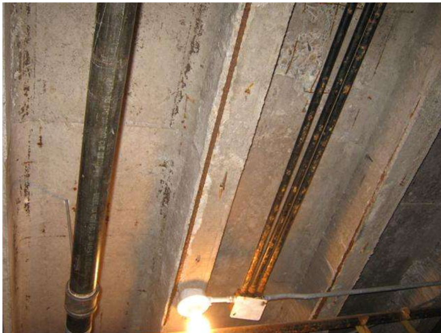
Cast in place concrete tee floor slab
