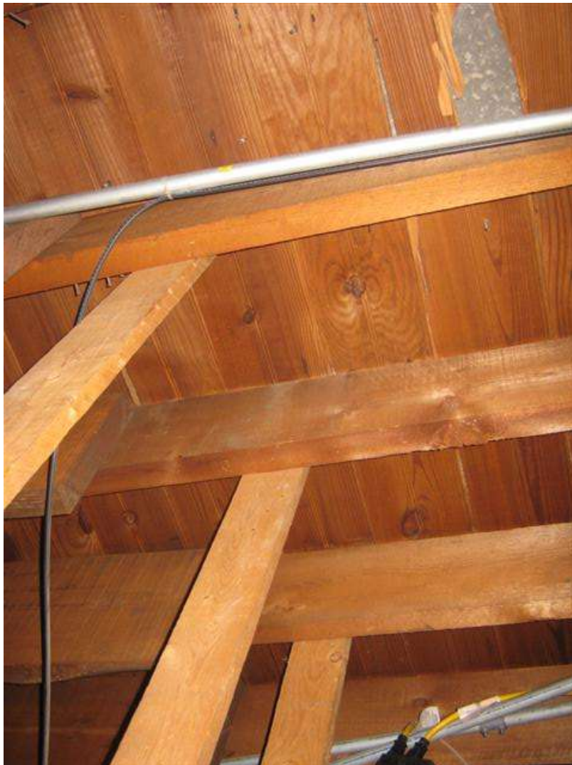
Wood roof joists and deck and supporting bearing walls
