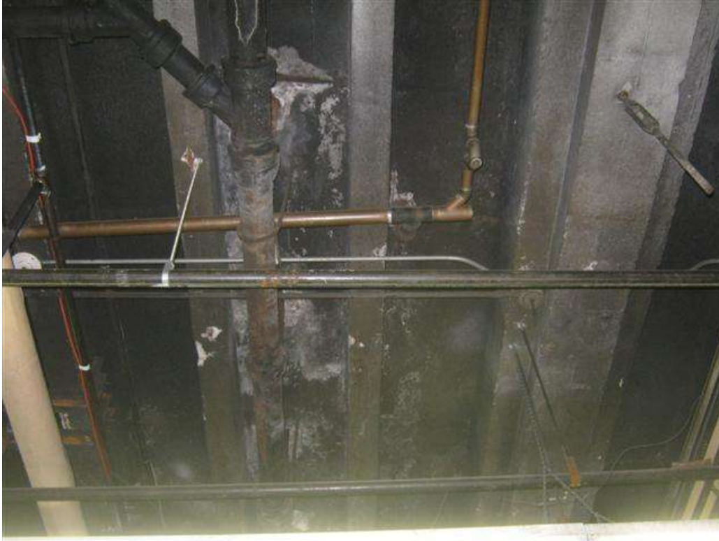
Cast in place concrete tee floor slab viewed from the Boiler Room
