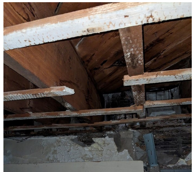
Figure 2 – Wood Framing Below Second Floor Classrooms
