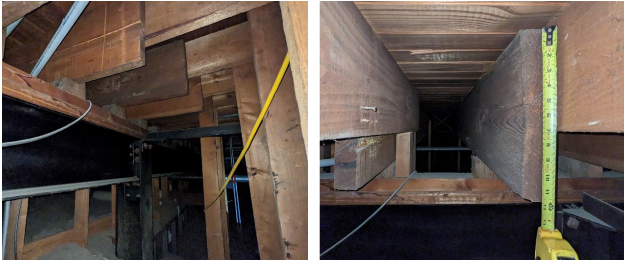
Figure 9 – Attic photos showing steel beam, column, and wood roof framing
