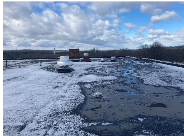
Roof, note exhaust fans
