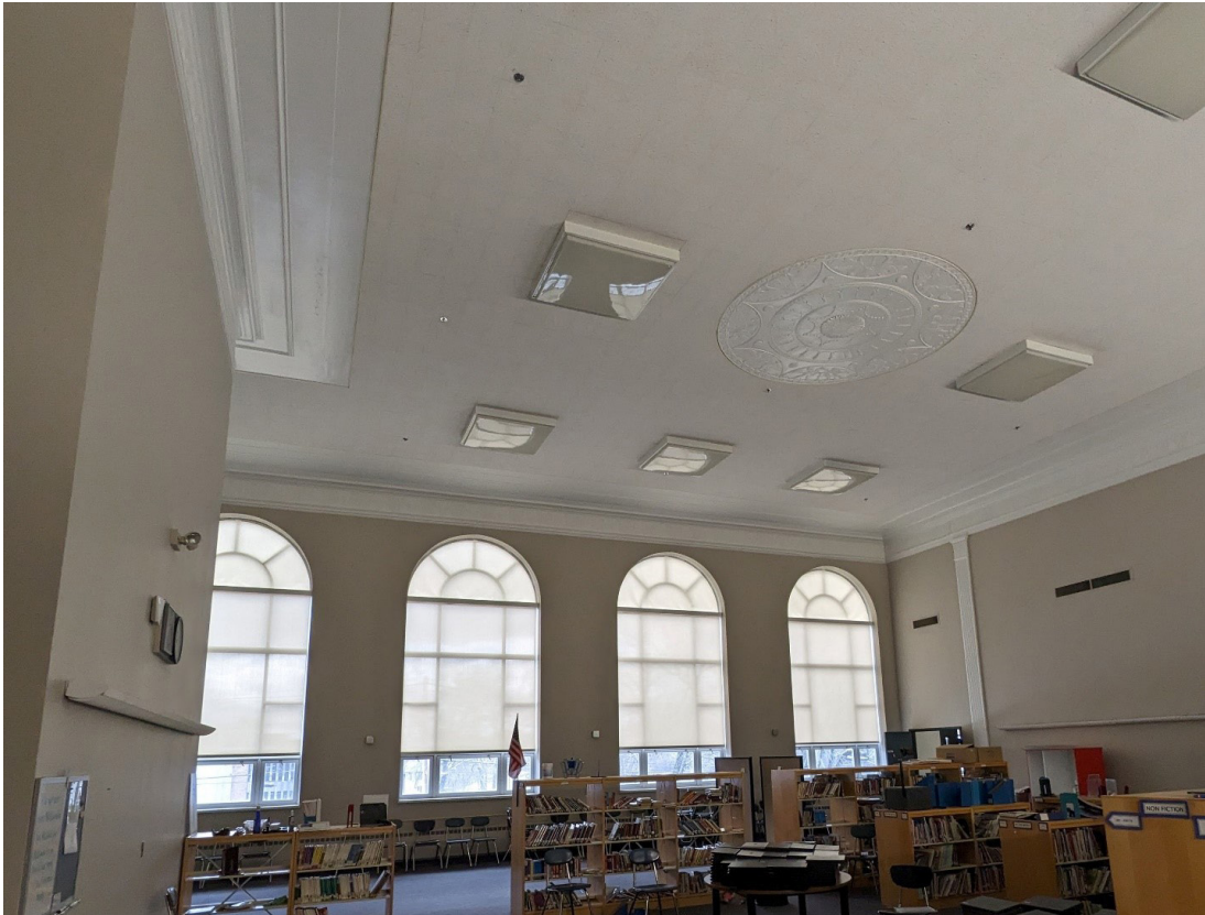
Figure 8 – Two-story library structure
