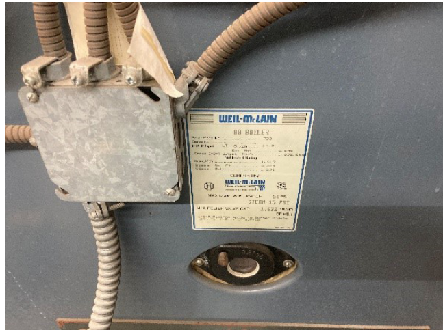
Boiler Nameplate
