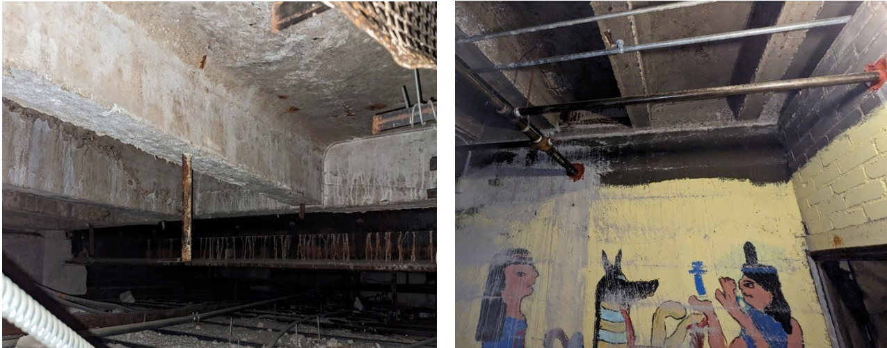
Figure 3 – Reinforced concrete rib-slab construction above kitchen and lower-level storage.
