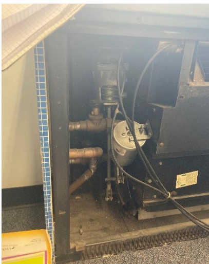
Typ. Heating UV, note piping and pneumatics
