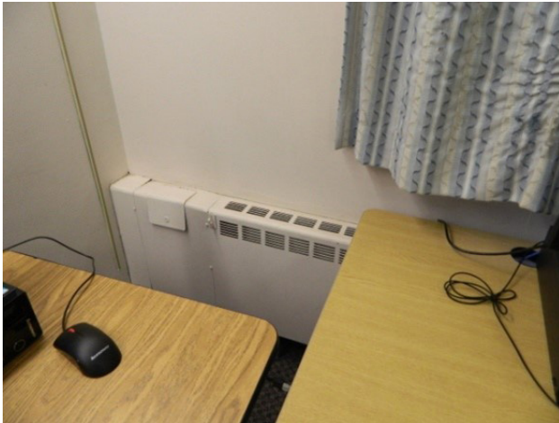
Typ. Finned-Tube radiation
