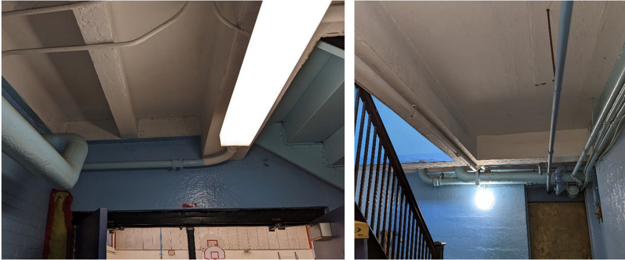
Figure 4 – Reinforced concrete beams and slab construction in stairwells.
