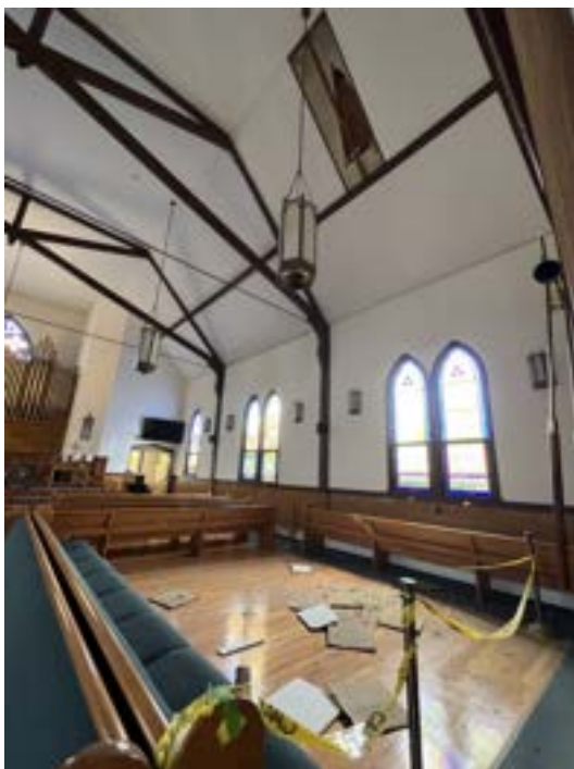
On July 1, 2023, a large section of ceiling tile failed leaving a large hole in the sanctuary ceiling.
