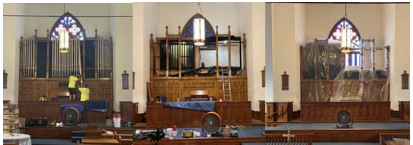
On September 11, 2023, the historic tracker organ in the sanctuary, installed in 1905, was partially disassembled—all exposed pipes removed—and the entire case covered in plastic to protect it from falling debris and dust.
