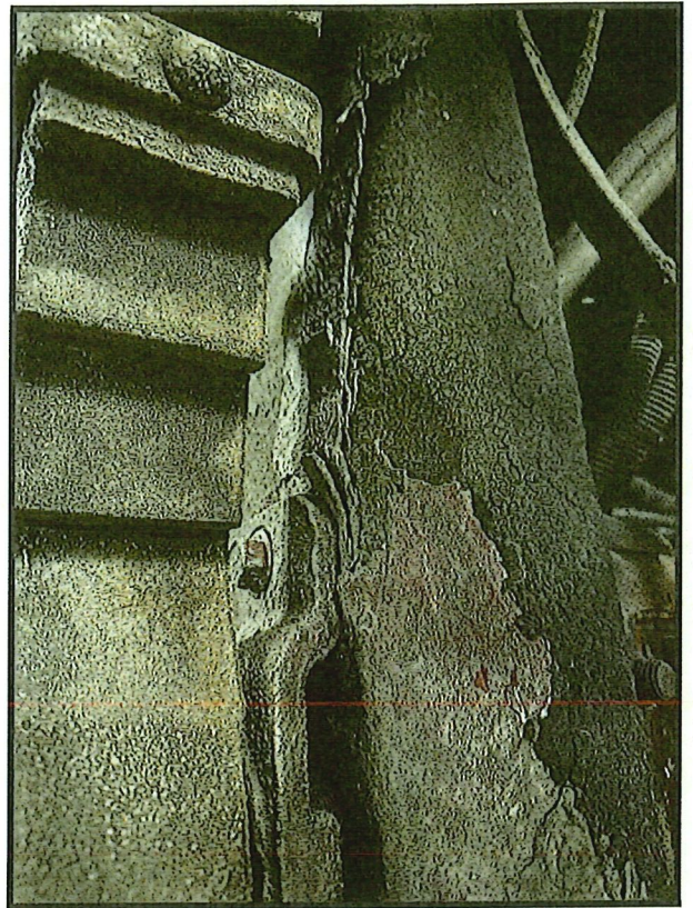
Frame Rail Corrosion with Delamination
