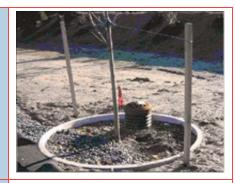
Other Subsurface Recharge Systems - Subsurface structures are underground systems that capture runoff and gradually infiltrate it into the groundwater through rock and gravel. There are several underground infiltration systems that can be installed to enhance groundwater recharge with the most common types including pre-cast concrete or plastic pits, perforated pipes, and galleys.
