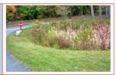
**Sediment Forebays** - A sediment forebay is a post-construction practice consisting of an excavated pit, bermed area, or cast structure combined with a weir, designed to slow incoming stormwater runoff and facilitate the gravity separation of suspended solids.
