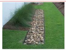
**Dry Wells** - small, excavated pits, backfilled with aggregate, and used to infiltrate uncontaminated runoff from non-metal roofs or metal roofs located outside the Zone II or Interim Wellhead Protection Area of a public water supply and outside an industrial site.
