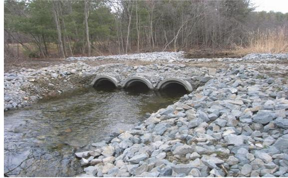
New stormwater management culverts installed at Dacey Recreation Area.
